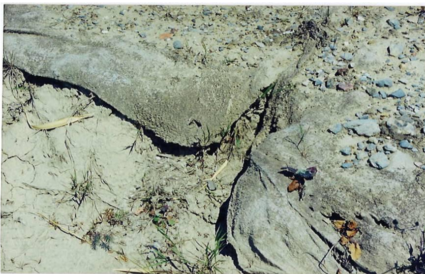
Fig. 2 Attempt to stabilize the dump Boşneag with textile fabric
